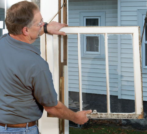
Remove old window sash and stops.
