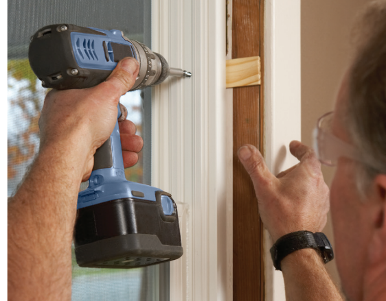
Fasten to existing frame, caulk and seal.
