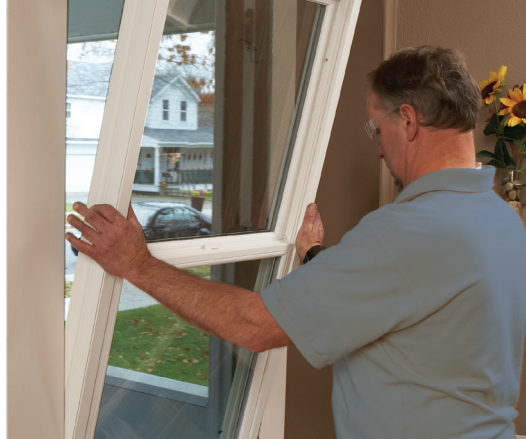
Insert new replacement window.
