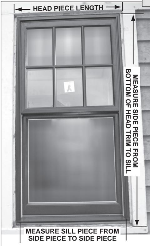
The head piece must be applied with a notch at each end. The side pieces are cut flat at the top and notched at the bottom. The sill piece is cut flat on both ends.
