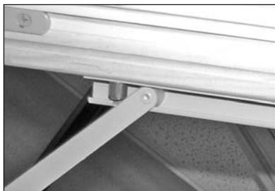
4. **For the split-arm operator**, use the crank handle to open the operator. Align the operator arm above the pin on the operator bracket. Push down on the operator arm to snap the arm onto the pin (**FIGURE 6**). Once the top and bottom hinge arms and the bottom operator arm are secured, the sash can be closed and locked.
