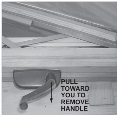
**NOTE:** To provide clearance for taking out the screen, remove sash crank handle by pulling it off its shaft (**FIGURE 1**).
