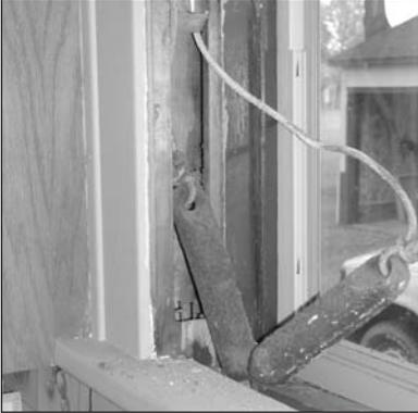
1. Cut sash cords and remove sash weights from both side jambs (**FIGURE 1**).
