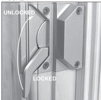
1. Sash is locked when lock lever is pulled down against the stop (**FIGURE 1**).
