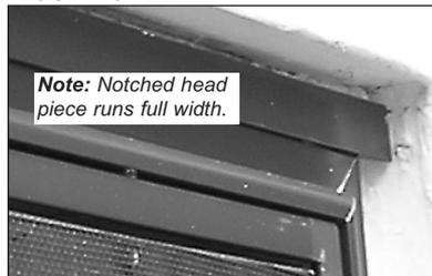
3. After trim is cut to size, remove sharp or rough edges.
