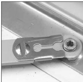
4. On a single-arm operator, open sash until operator is in the mid point of the operator track. There is a notch in the underside of the operator track that will allow the roller on the end of the operator arm to be released from the track by pushing down on the operator (FIGURES 6 & 7). Use the crank handle to close the operator to get it out of the way.
