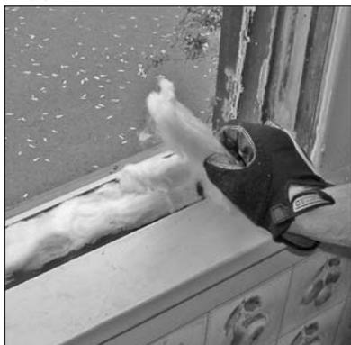
5. Insulate space between angle support bracket and stool with fiberglass insulation (FIGURE 7). **Do not over pack insulation.**
