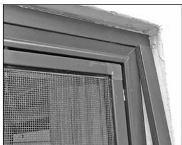
5. Measure, cut and install side pieces. Side trim runs from bottom of head piece to old sill and is flat at the top and notched at the bottom (FIGURES 7 & 8).
