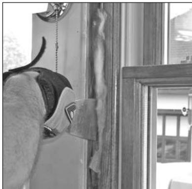
13. Loosely insulate between the new window jambs and the old window frame with fiberglass insulation (**FIGURE 13**). Low expansion foam insulation, specifically rated for window and door application, may be used instead of fiberglass.
