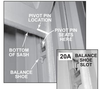
7. After pivot pins are fully engaged in balance shoes, tilt or push the top of the sash up and away from you (FIGURE 21) until both tilt latches snap into the side jambs. Tug gently inward on top of lower sash to check tilt latch engagement.
