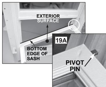
4. With one side of sash angled up (FIGURE 19), place pivot pin so it sits on the top of the balance shoe in the side jamb (FIGURE 20). Lower opposite side of the sash, so that its pivot pin is above opposite side balance shoe (FIGURE 20A).
