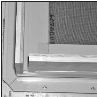
FIGURE 2 PVC JAMB EXTENSION
