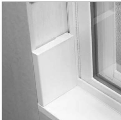
FIGURE 3 PVC JAMB EXTENSION
